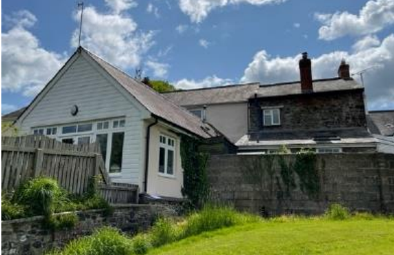
Image of rear wing facing south-east
