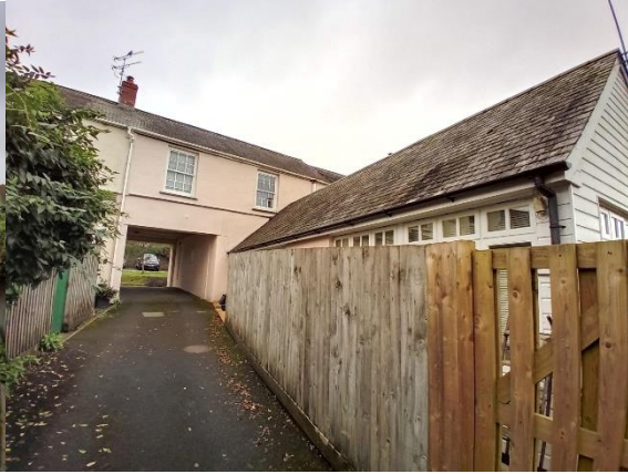
Image of rear wing facing south-west
